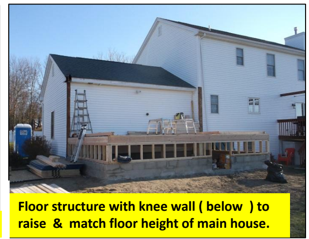
Excavate , foundation, slab & backfill complete.
