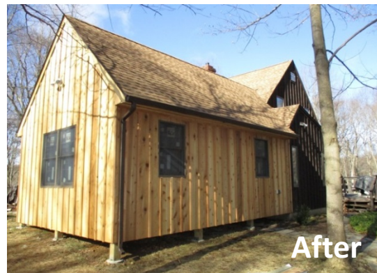
Completion of exterior framing ( cathedral ceiling ) windows , matching vertical cedar siding & roof shingles / gutters .
