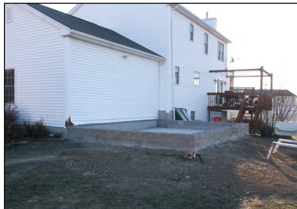
Excavate , foundation, slab & backfill complete.
