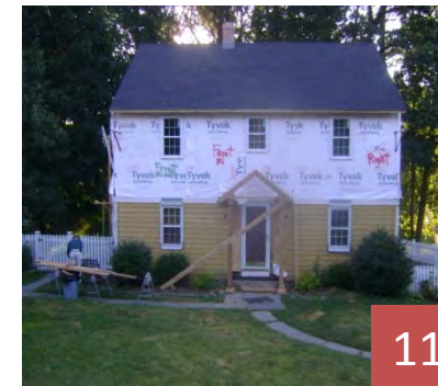
11. End of next working day , roof completely sheathed & shingled . Next day chimney raised & windows installed.
