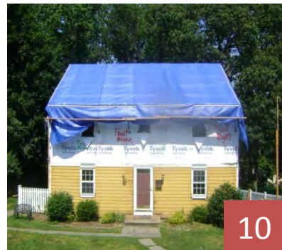
10. End of day , roof partially sheathed and completely covered with a tarp.
