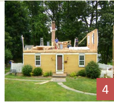
4. Started to erect pre-built walls by 12:30 pm.
