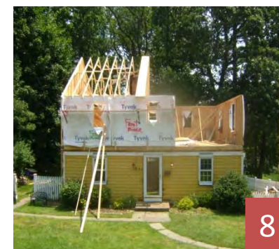
8. Pass up all pre-built roof trusses through open wall area ( See front , right side ).
