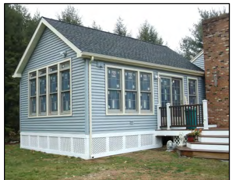
Exterior complete, roof shingles , windows , door, siding , gutters, skirt.
