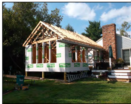
Walls erected, roof 50 % framed.
