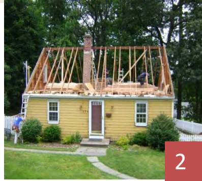
2. Removal of existing roof. See new exterior walls stored & stacked on attic floor.
