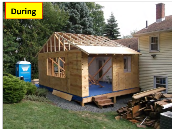
Walls & trusses erected
