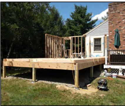
Support post , floor structure , start walls.
