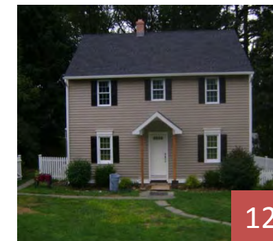
12. Finishing touches , vinyl siding , gutters & shutters.
