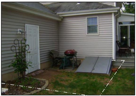
1) Before picture . Proposing to build a rear addition with full bathroom & bedroom. ( see dotted lines )
