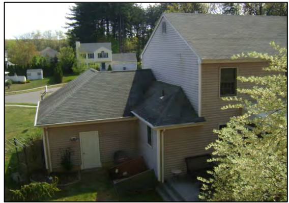
3) Before picture , rear elevation, note variety of existing roof lines.
