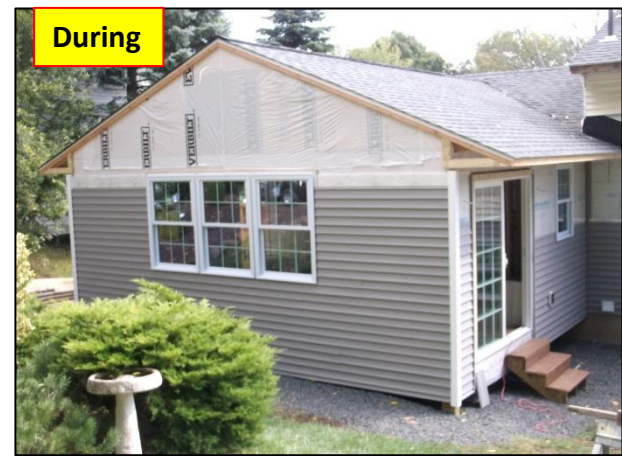
Roof shingled , windows / doors , start siding
