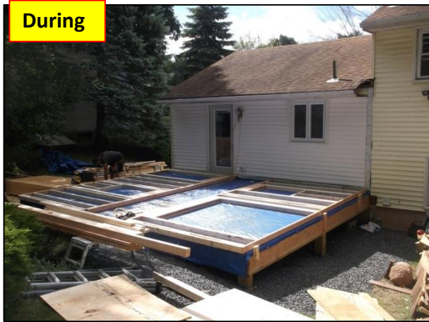
Footings excavated & poured , floor framed
