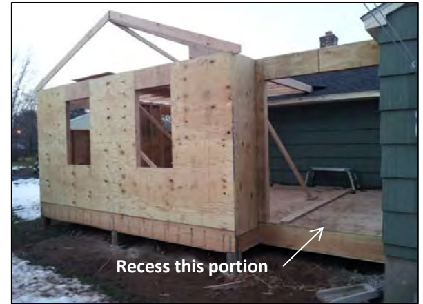
3) Floor sheathing complete, constructing and raising exterior walls in progress.
