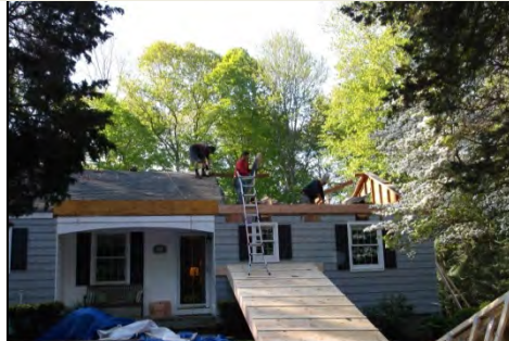
10:00 AM, roof 75% removed
