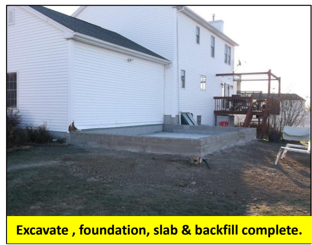
Floor structure with knee wall ( below ) to raise & match floor height of main house.
