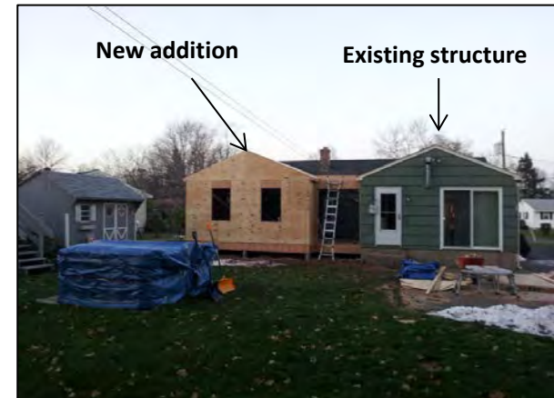
4) Finishing shell & shingling roof in progress.
