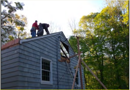
8:00 AM, roof 25% removed
