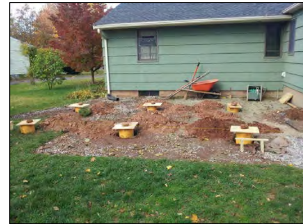
1) Addition on piers, Excavate & pour concrete footings.
