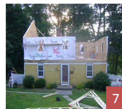
7. End of day , all erected exterior walls braced and end gable erected . See roof trusses on ground.
