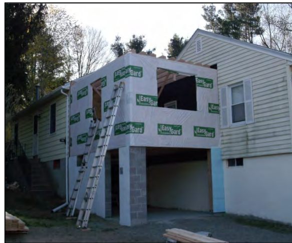
During ( shell , shingles & windows )
