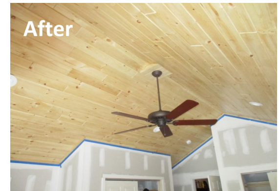
Completion of interior drywall, trim and ceiling planking
