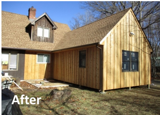
Completion of exterior framing ( cathedral ceiling ) windows , matching vertical cedar siding & roof shingles / gutters .
