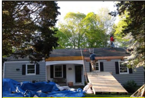
7:00 AM, start removing roof
