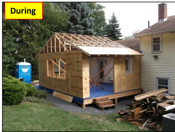
Walls & trusses erected
