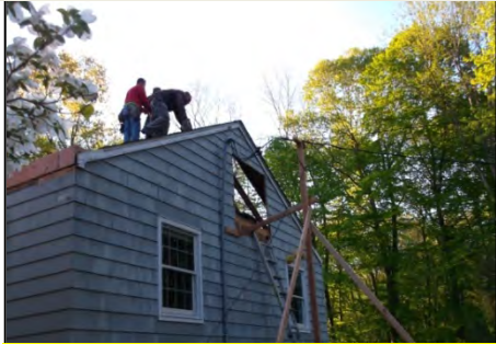
8:00 AM, roof 25% removed
