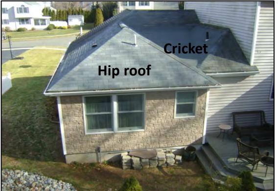
6) Completed roof , rear elevation view. Solution to complicated roof lines.
