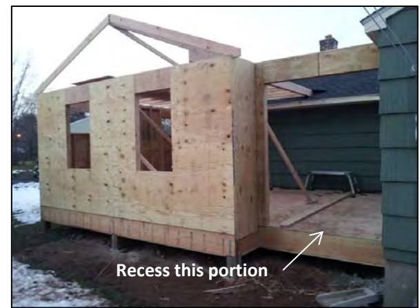
3) Floor sheathing complete, constructing and raising exterior walls in progress.
