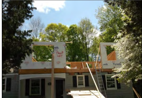
2:00 PM, Walls up, carry trusses.
