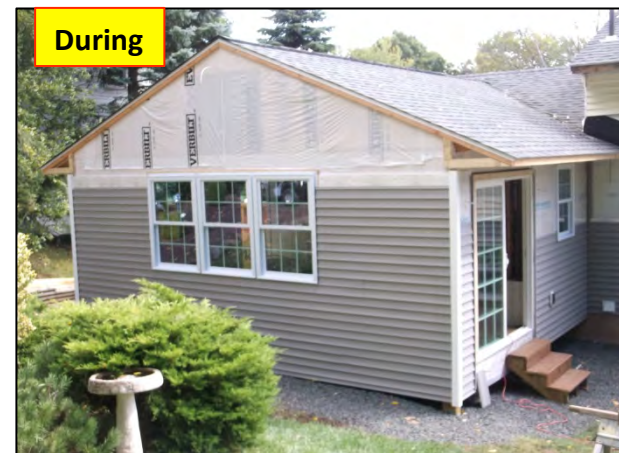
Roof shingled , windows / doors , start siding
