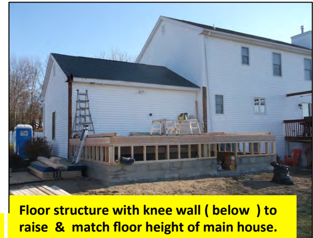
Excavate , foundation, slab & backfill complete.
