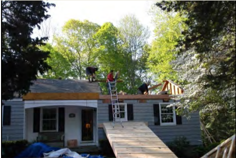
10:00 AM, roof 75% removed
