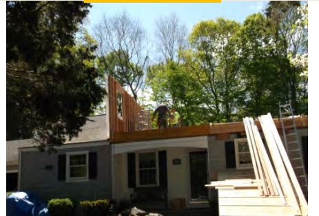
12:00 PM, start raising walls
