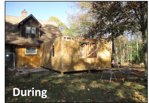
Erecting exterior walls
