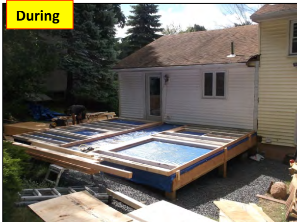
Footings excavated & poured , floor framed
