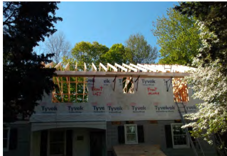
5:00 PM, last wall & roof trusses
