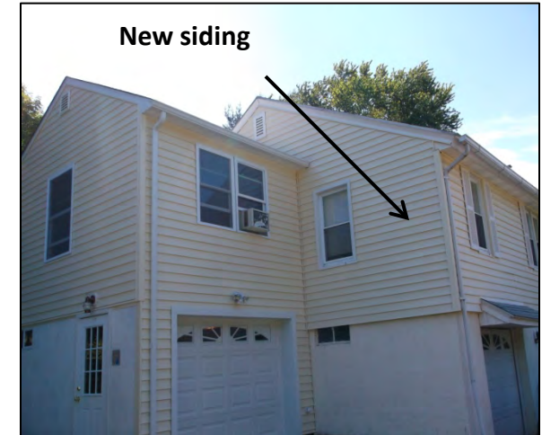
Completed ( siding , gutters , doors )
