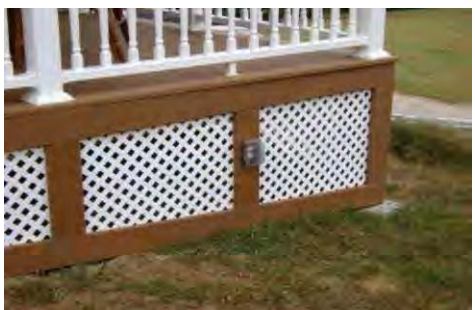
Bottom Skirt with electrical outlet
