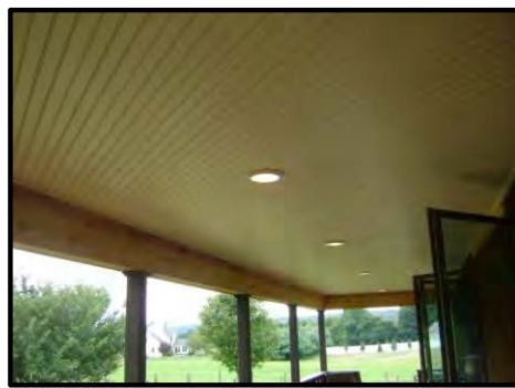
Diagonal Vinyl wainscoting ceiling
