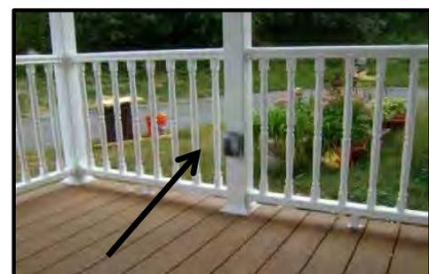
**Electrical outlet inserted Into hollow post**
